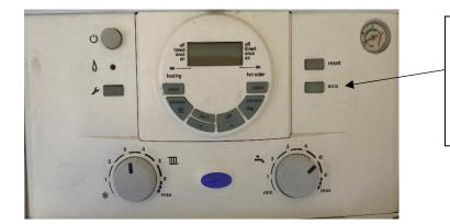
On some combi boilers there is an "Eco" button which when pressed stops the pre heating function which will use more gas and just reduces the cold water run off.
