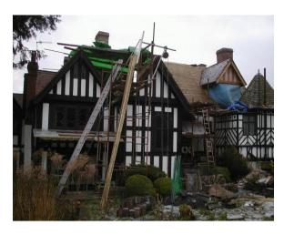
The rotted pine timbers of structurally unsound Victorian additions were replaced by oak framed panels backed with Kingspan and faced with lime mortar.
